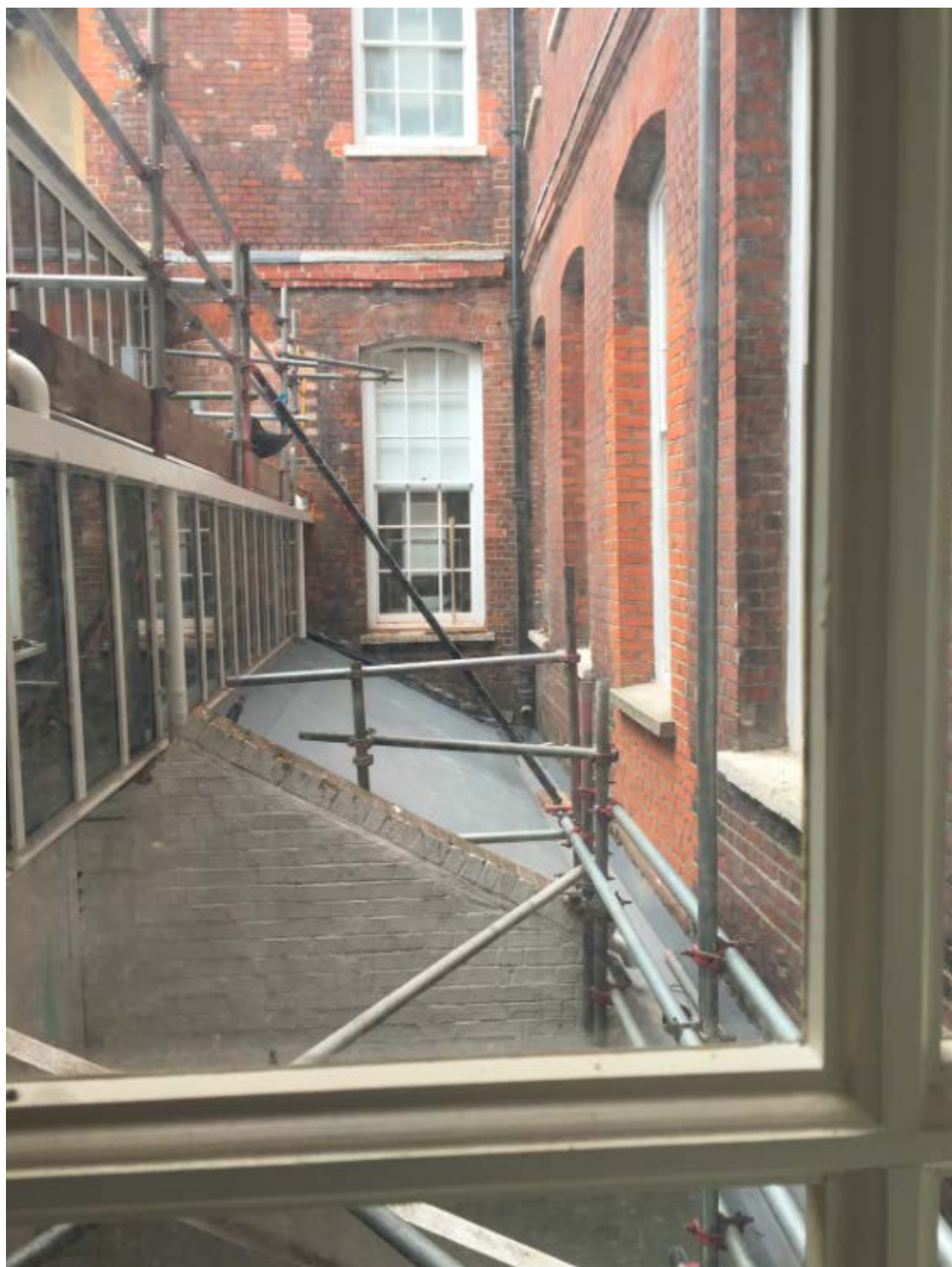
View from bathroom window of Flat 1, 43 King Street
